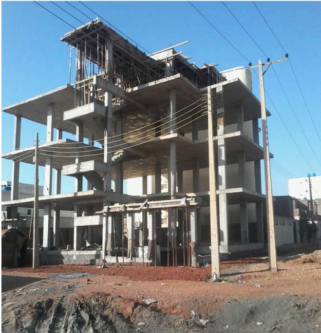
Reinforced-concrete frame under construction
