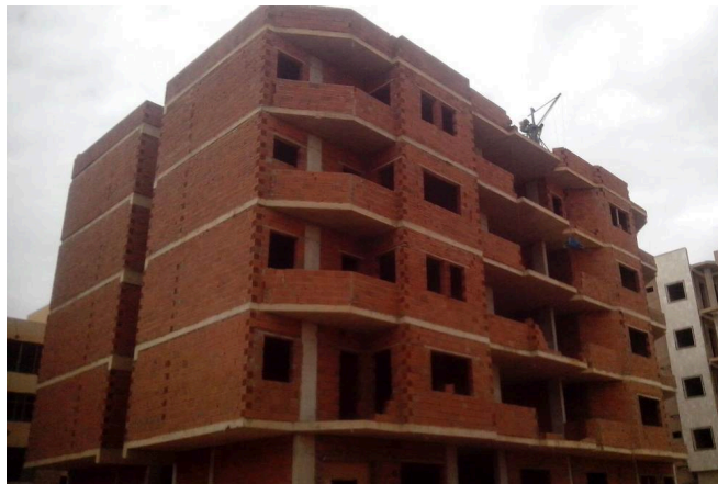
RC frame complete with brick masonry
