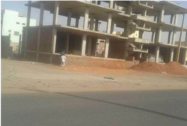
Concrete structure under construction
