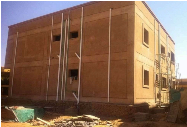
Masonry & external finishing
