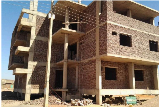
Brick masonry works
