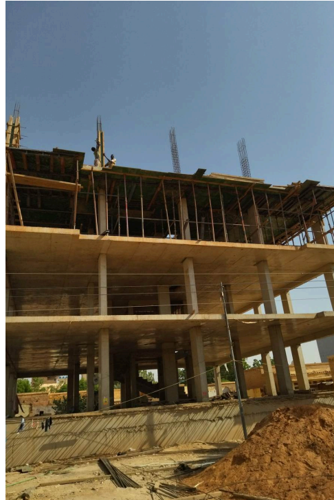
Concrete frame under construction
