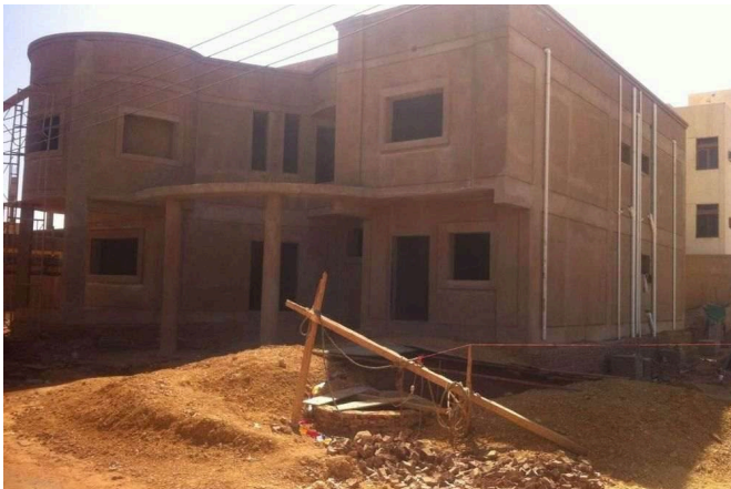
Structure under construction
