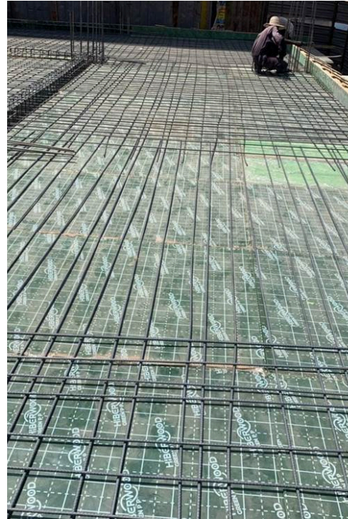
Foundation reinforcement
