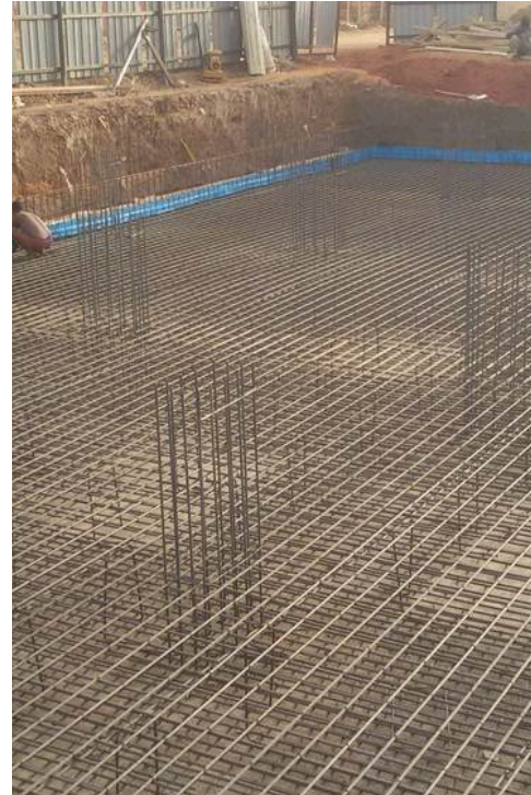
Raft reinforcement
