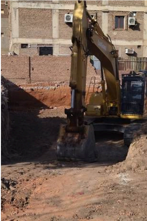
Excavation & foundation works
