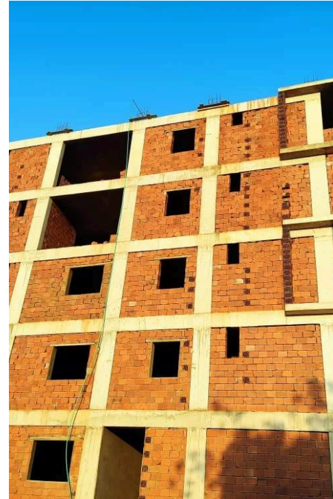
Masonry works — full height
