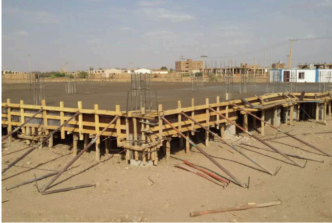
Foundation formwork — start of works
