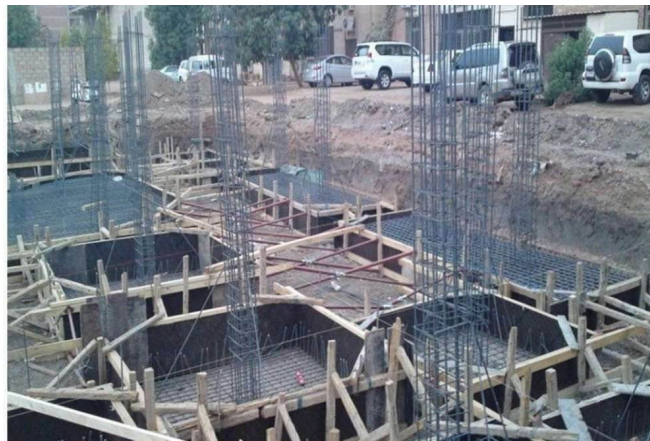
Foundations under construction
